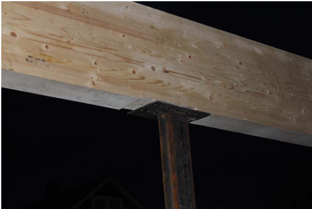
26. The column is placed under beam.
