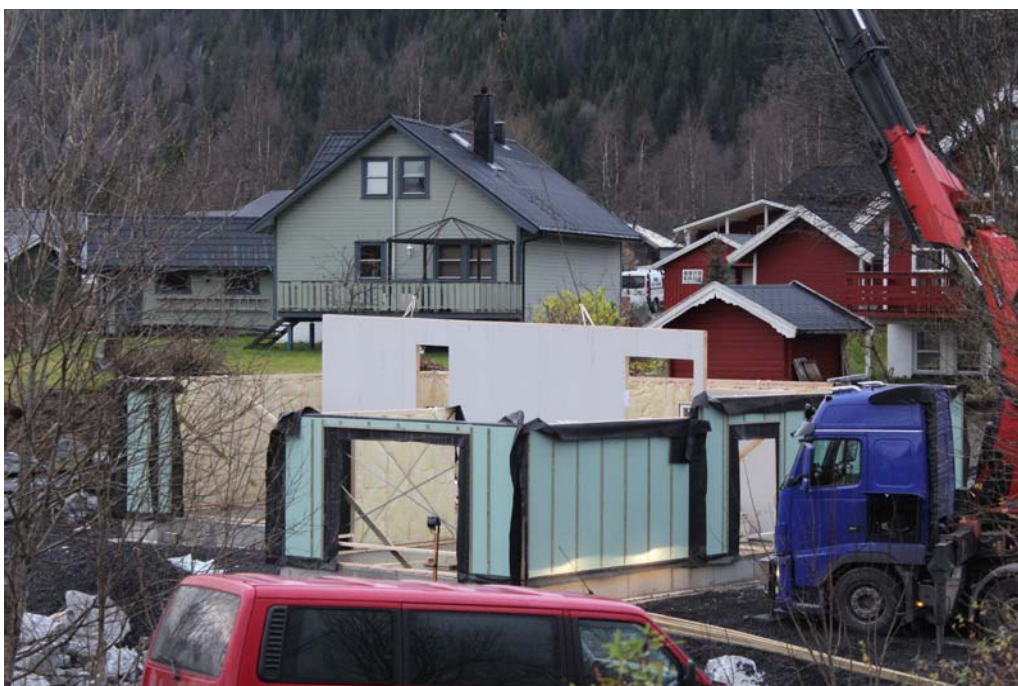
16. Load bearing wall Element no.9 positioned for placement.
