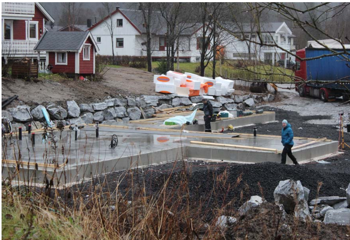
1. Here is concrete plate on the ground ready for mounting of the house.
