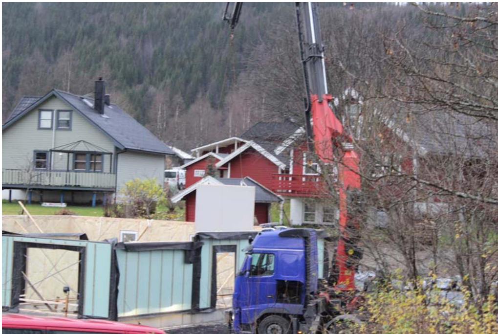
14. Load bearing wall Element no.10 is placed. Poor logistics made the Glulam Beam 7 and 8 as well as load bearing wall Element no.9 not available and could not be installed in right order.
