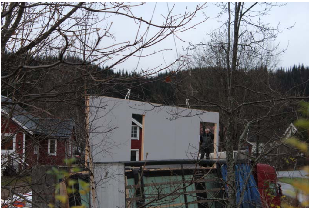
15. Load bearing wall Element no.9 arrived from truck.
