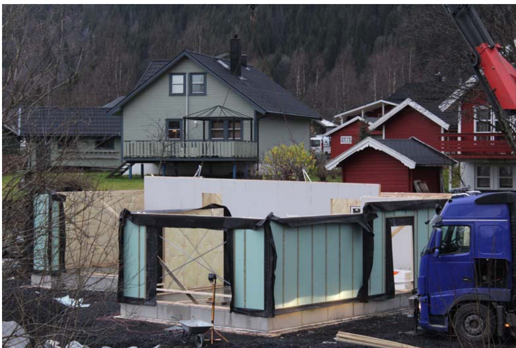
17. Load bearing wall Element no.9 is placed.
