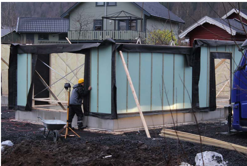
13. Element no.6B is placed.
