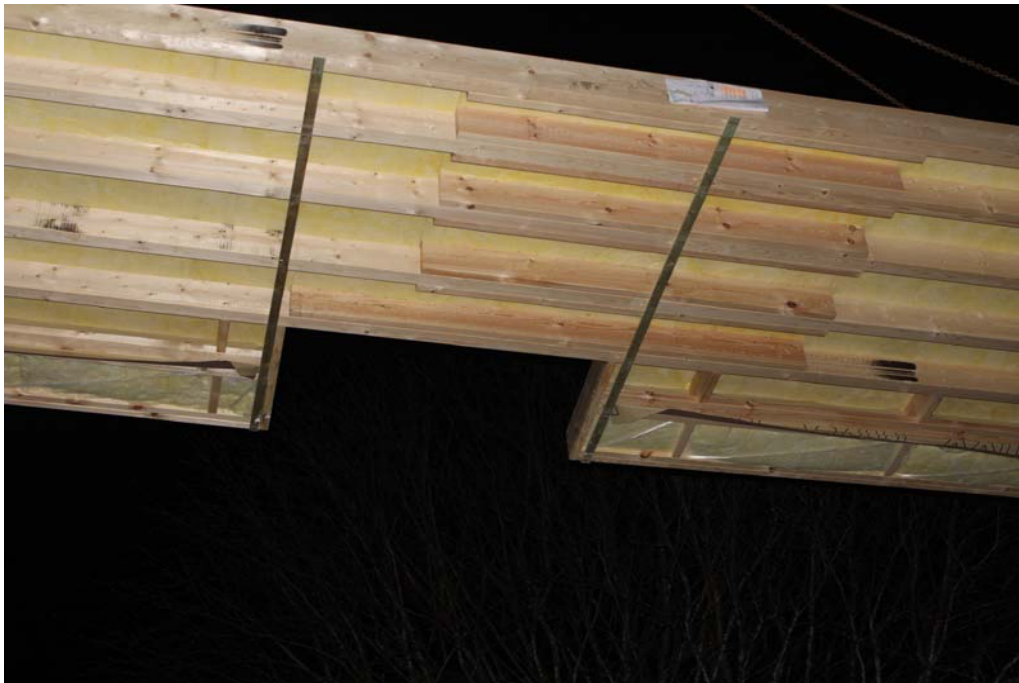
36. Floors Element no.11 in the air, recess is a balcony-bumps to be installed.
