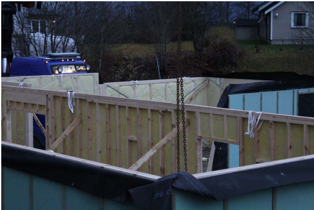
20. Here shows the load bearing wall with vertical stud spaced 30cm c/c in order to carry the 550 kilogram snow load for the place.
