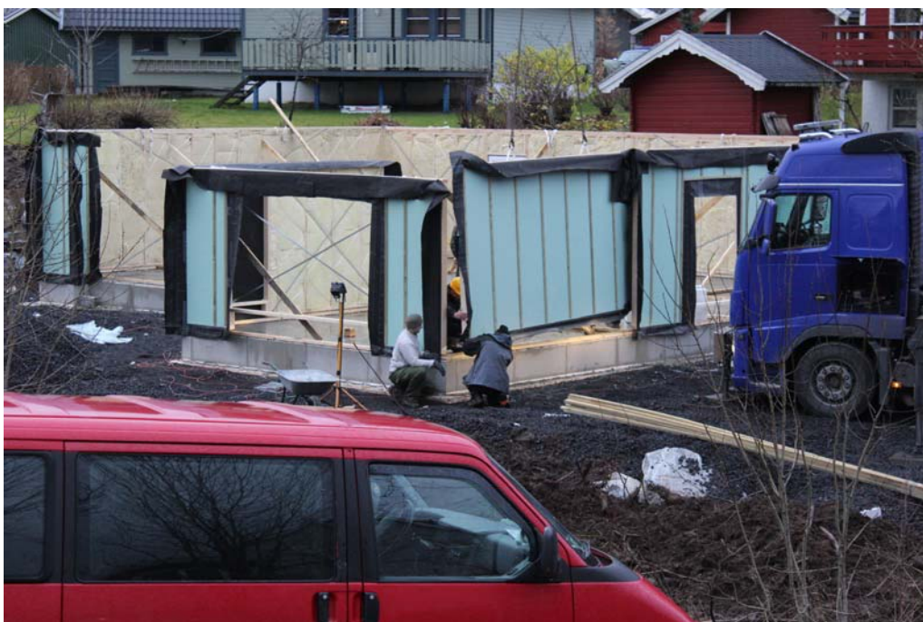
12. Element no.6B is positioned.
