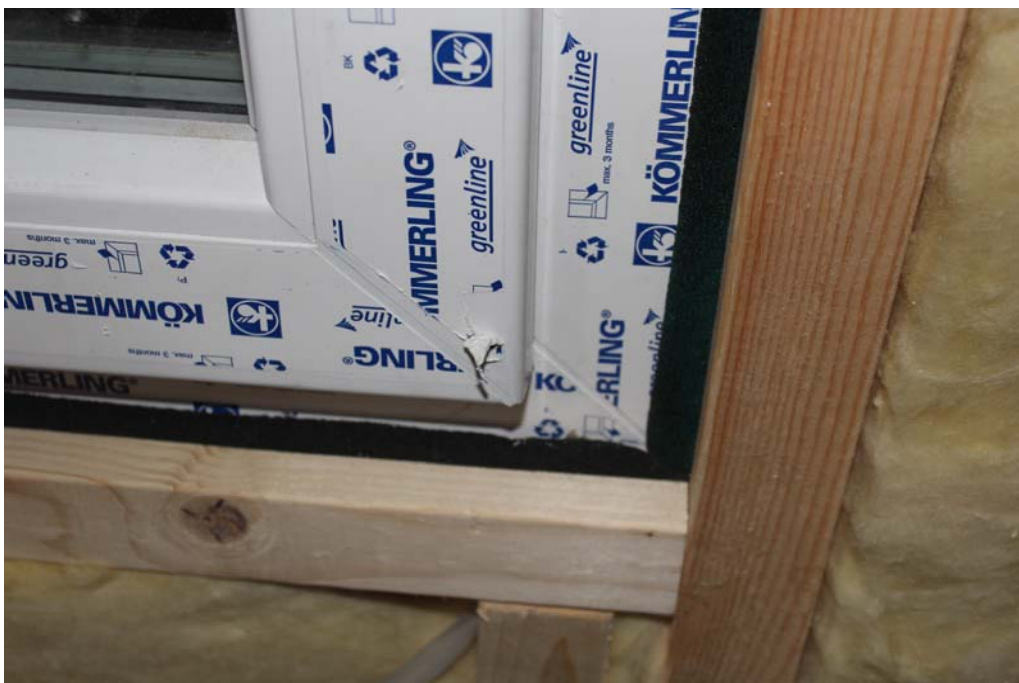
27. Special windows Kömmerring white interior and gray exterior inset into the wall with special bands approved by the Passive House Institute in Stuttgart for maximum sealing over the long term.
