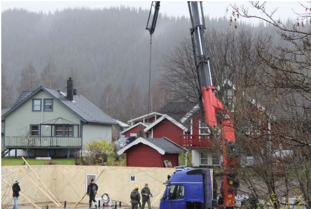
5. Crane deliver element no.2
