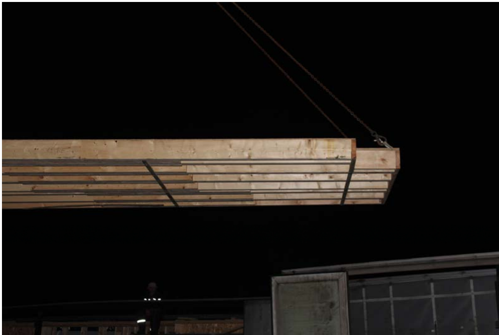
32. Unnecessary temporary storage of elements.
