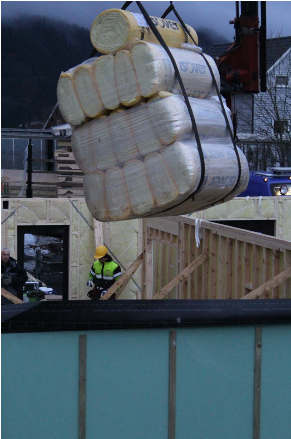
19. The hoisting of insulation while the workers are relaxing.
